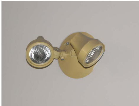
Illustration 12: Remote emergency light
