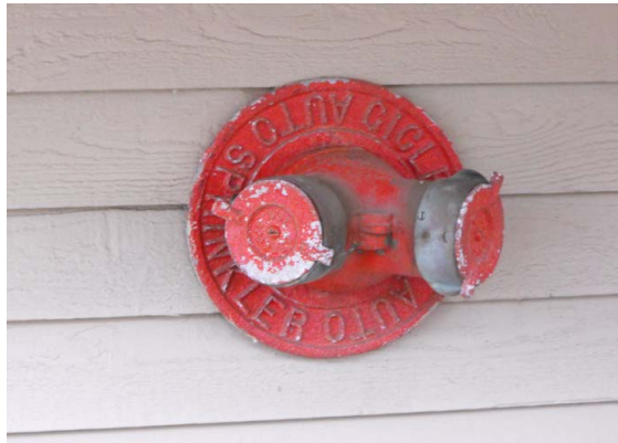
Illustration 7: Fire Department Connection
