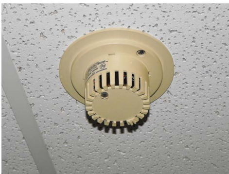
Illustration 13: smoke detector
