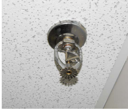
Illustration 14: Sprinkler head
