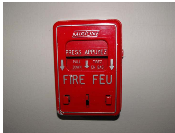
Illustration 10: Fire Alarm pull station
